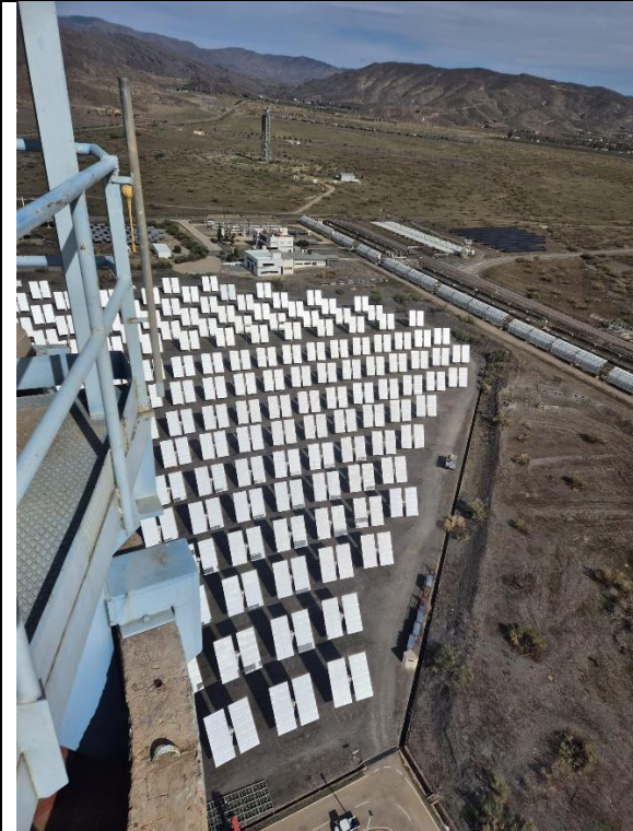
Fig. 2 Image taken from the top of the PSA's CESA-1 tower, showing part of the heliostat field.
